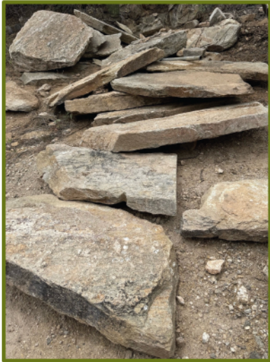
Original steps washed away in the flood of 2006
