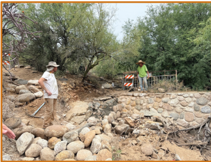
The new dam steps begin to take shape
